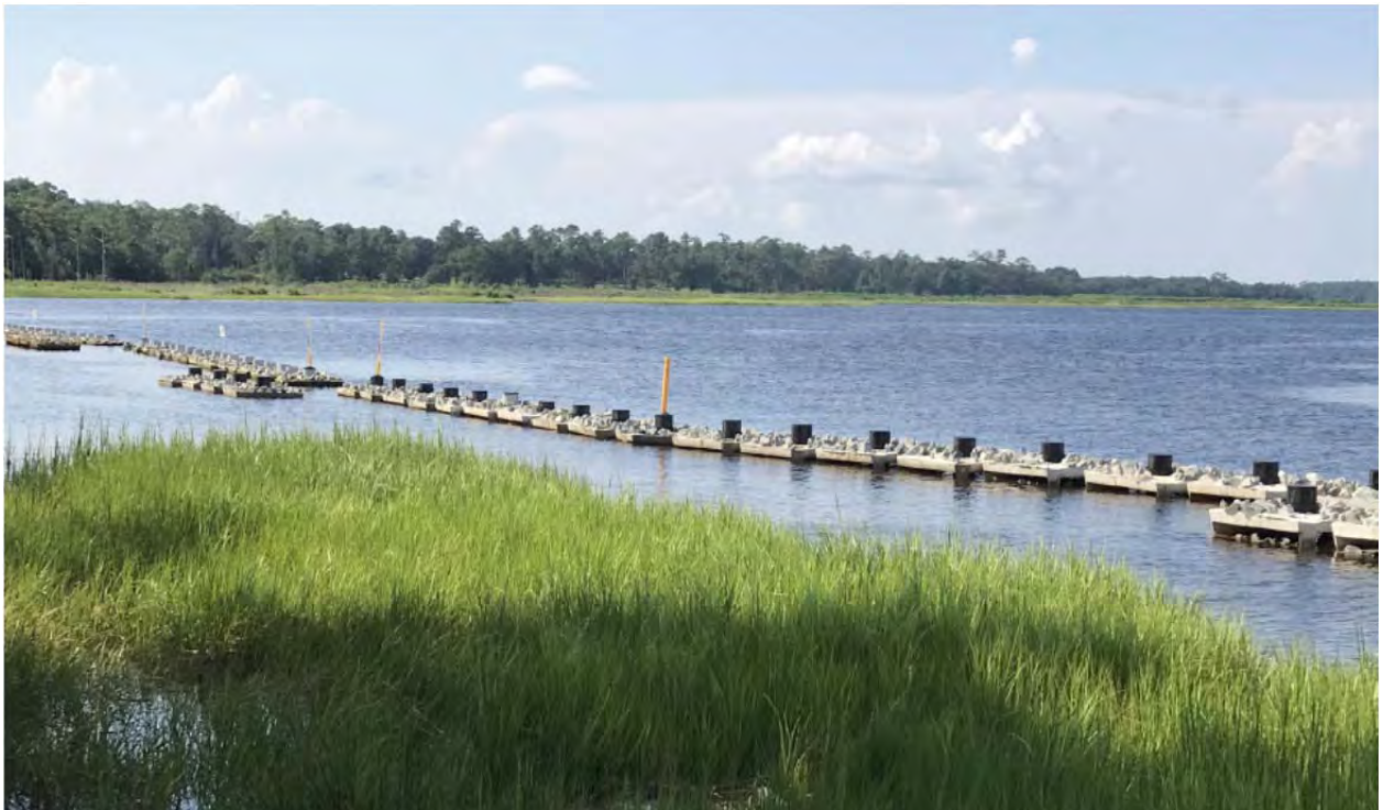
Figure 34 Example of Reef Maker Wave Attenuation Structure
