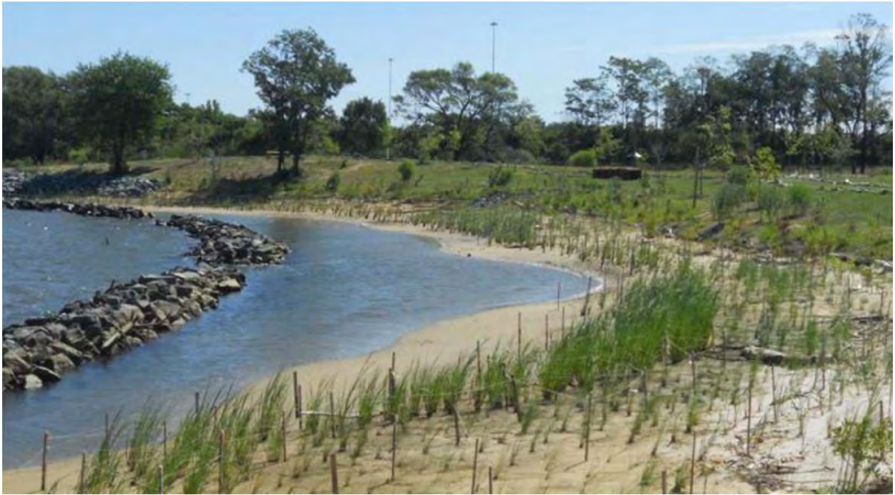
Figure 33 Example of Rock Sill Used for Shoreline Protection
