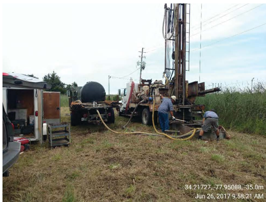
Monitoring well drilling at Site #1 – Front Street
