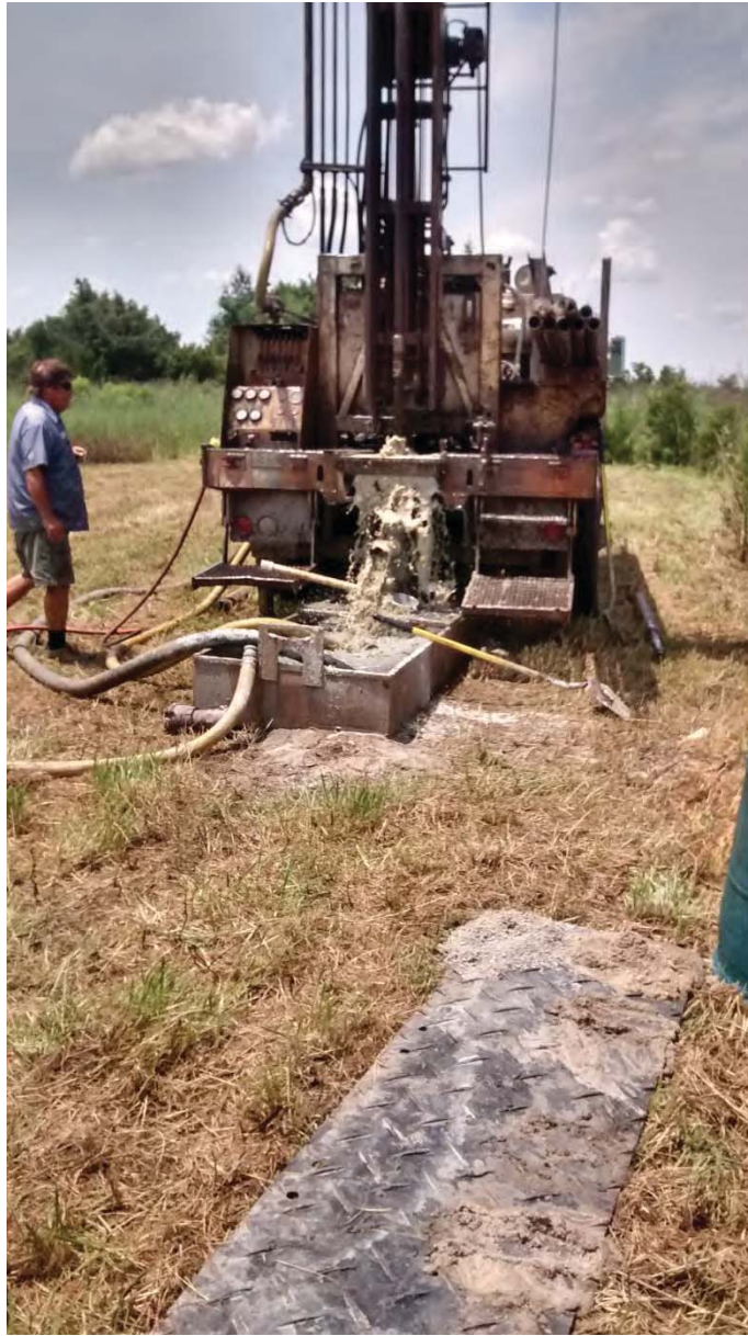
Air-rotary drilling of the Peedee Aquifer monitoring well, Site #1 – Front Street
