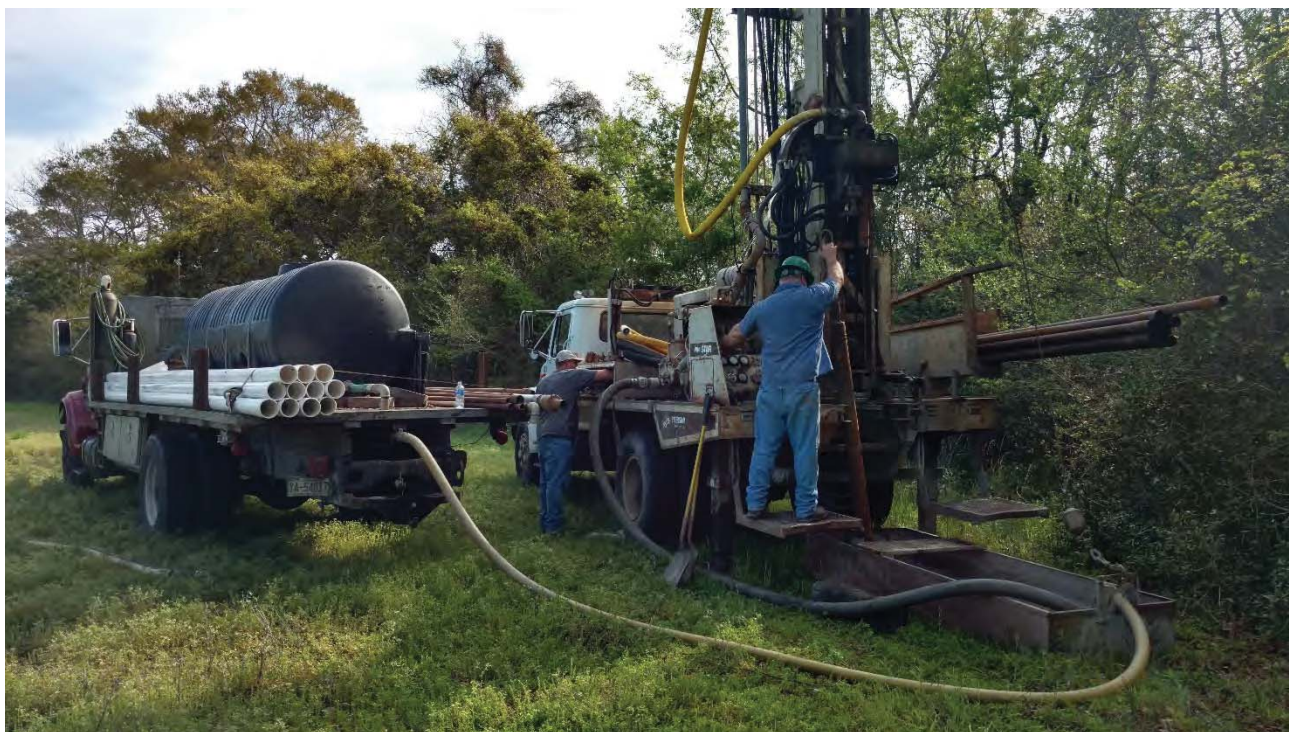
Monitoring well drilling at Site #3 – Southport
