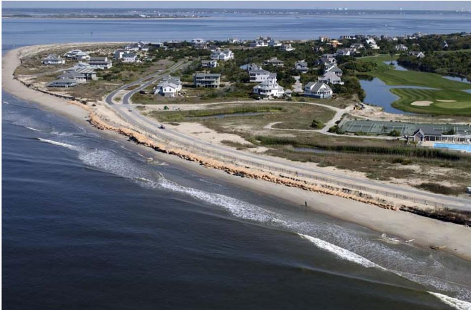
**Figure 2.8 Sand Bag Revetment along South Bald Head Wynd, April 2003.**
