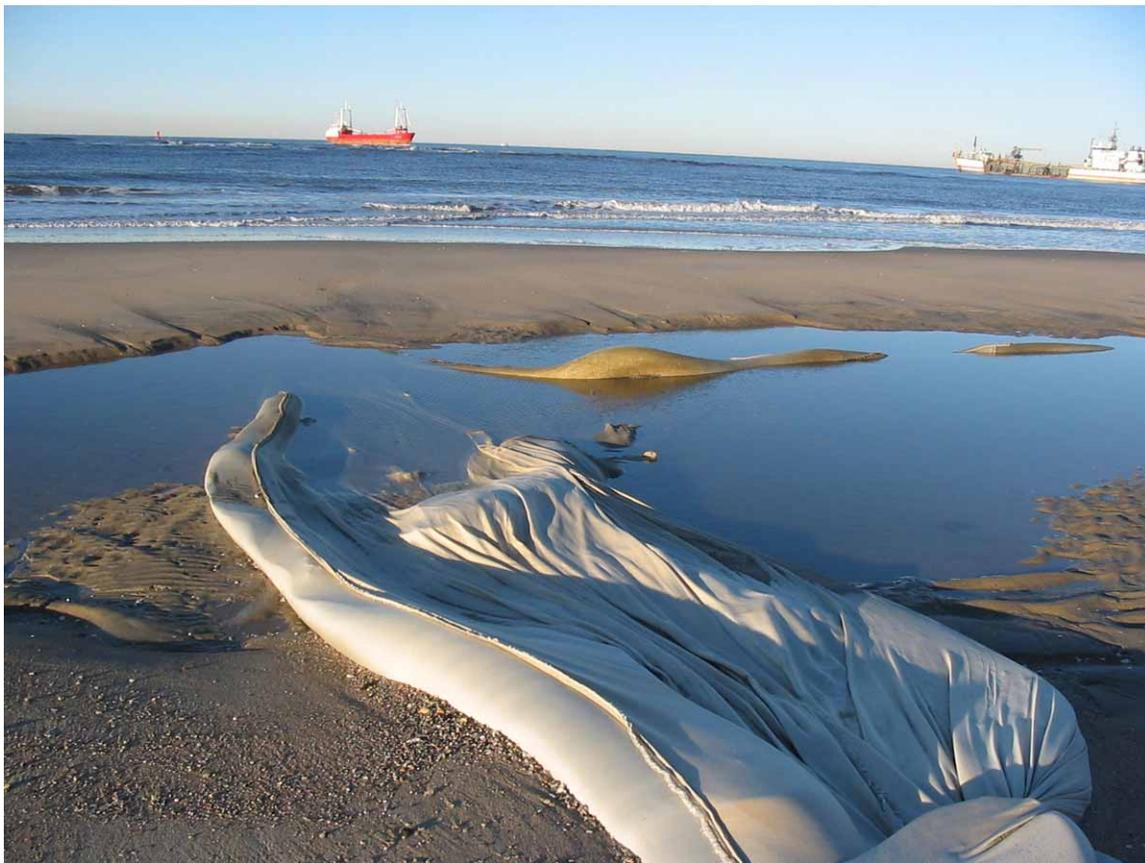
**Figure 4.10 The Remains of a Geotextile Groin near the West End of the Groin Field on 31 December 2003.**
