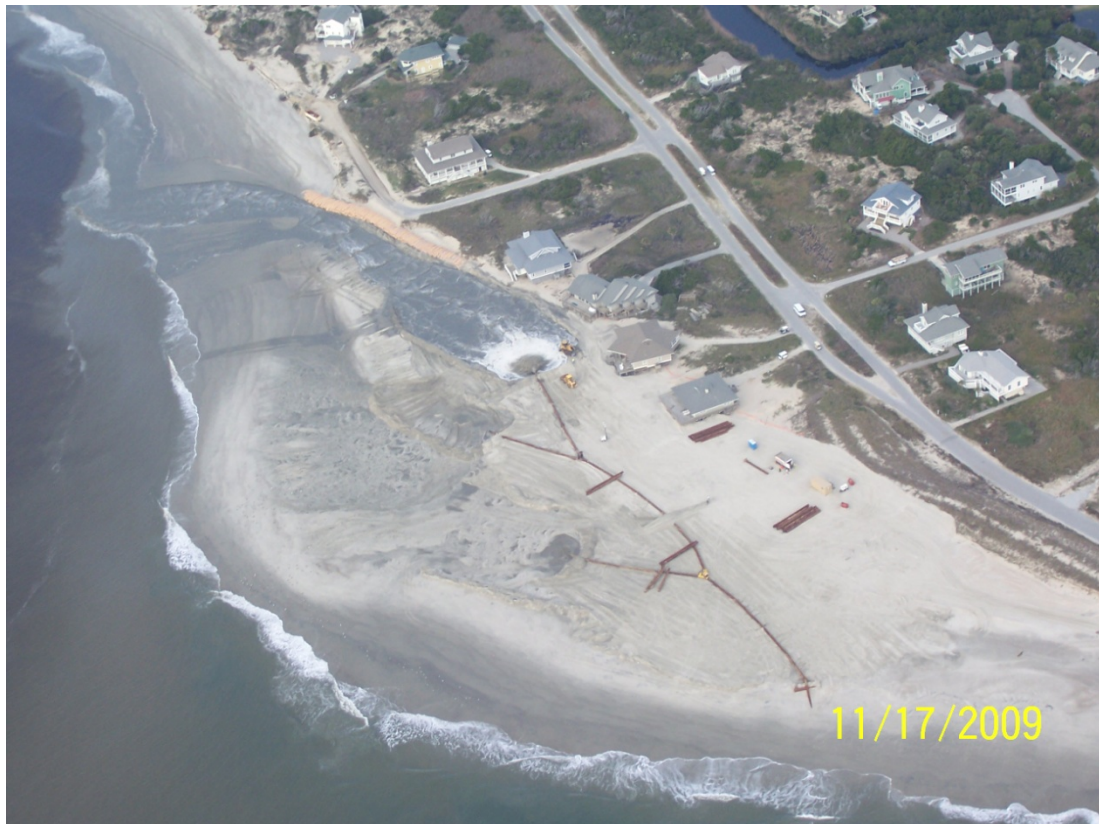
Figure 2.5 Start of the 2009-2010 local Beach Disposal Project along Bald Head Island, November 2009 (Courtesy of Village of Bald Head Island)
