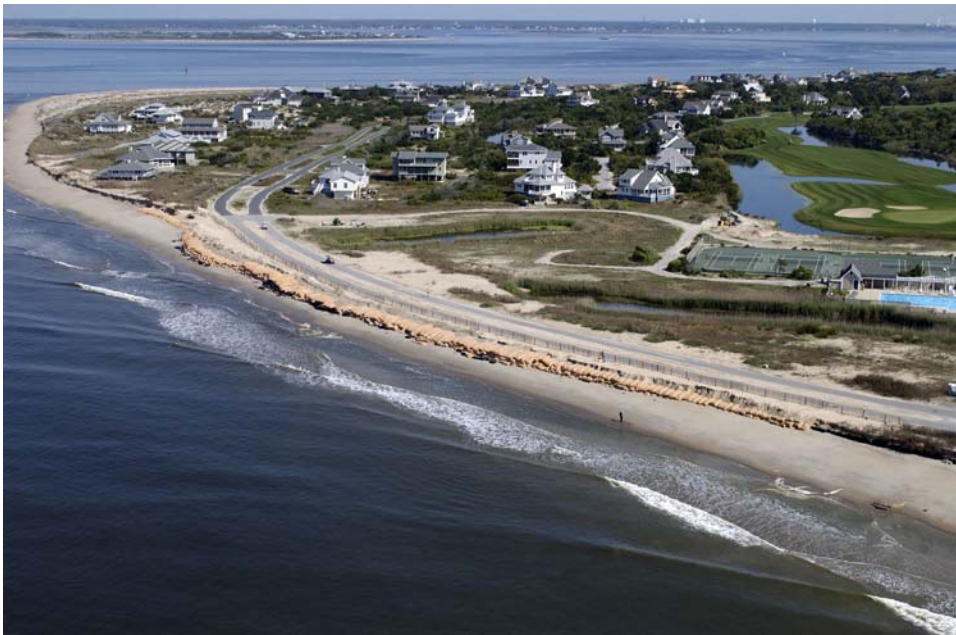
Figure 2.3 Sand Bag Revetment along South Bald Head Wynd, April 2003.
