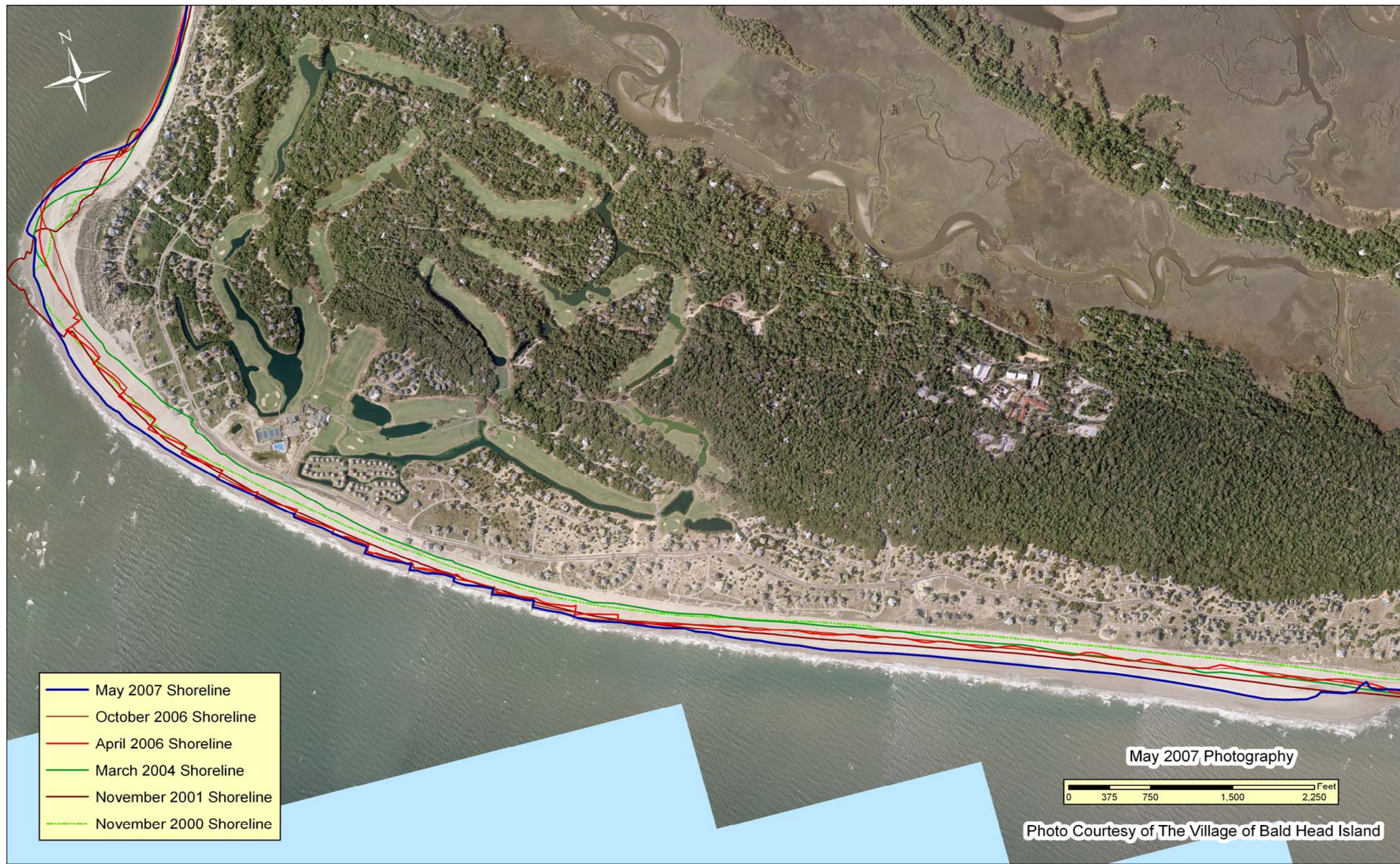
Figure 4.13. Shoreline Comparison: Pre and Post groin field reconstruction and beach disposal
